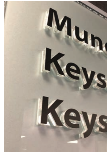
Example of letters mounted on the outside of tempered glass.
